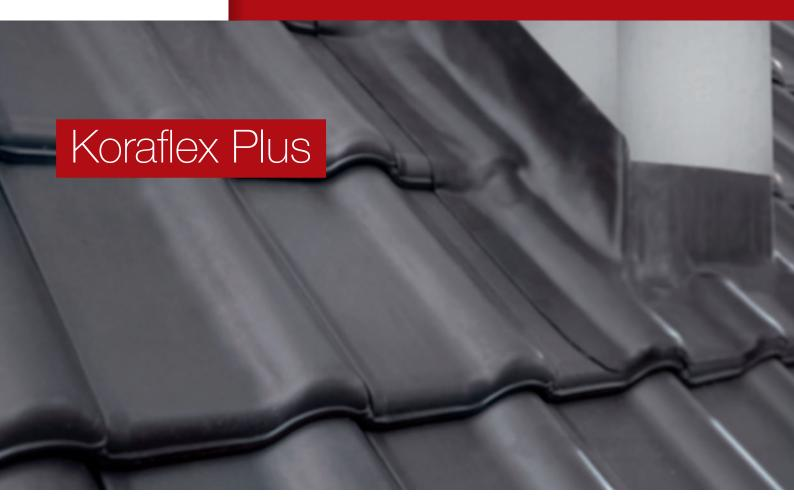
Malleable, durable lead-replacement flashing solution. Available in colours to match lead or to complement roof tile colours.
